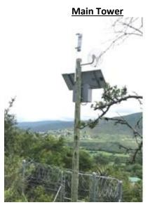
As seen in the picture above, our main signal is coming from our tower we had put up at the beginning of the year. The signal gets sent down to the computer lab. It is from the computer lab where the signal then gets bridged across the campus using the exterior access points.
