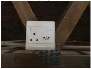
As seen in the picture above, we pre-installed plugs into the ceilings to provide power to all the cabinets. These plugs were routed back to the main DB board. They were labelled and installed with a trip switch. A COC certificate was provided.
