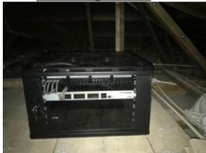
As seen in the picture above, all the cabinets were installed in the ceilings for safety. Since there were no servers in these cabinets, we used high temp graded switches in the ceilings. We also used outdoor network cables with a higher UV index rating. These cables also include an earth cable to protect against lightning.
