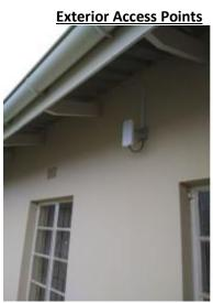
As seen in the picture above, we installed exterior AP's to bridge the signal across the campus. Each highlighted building has an exterior AP as well as interior Aps.
